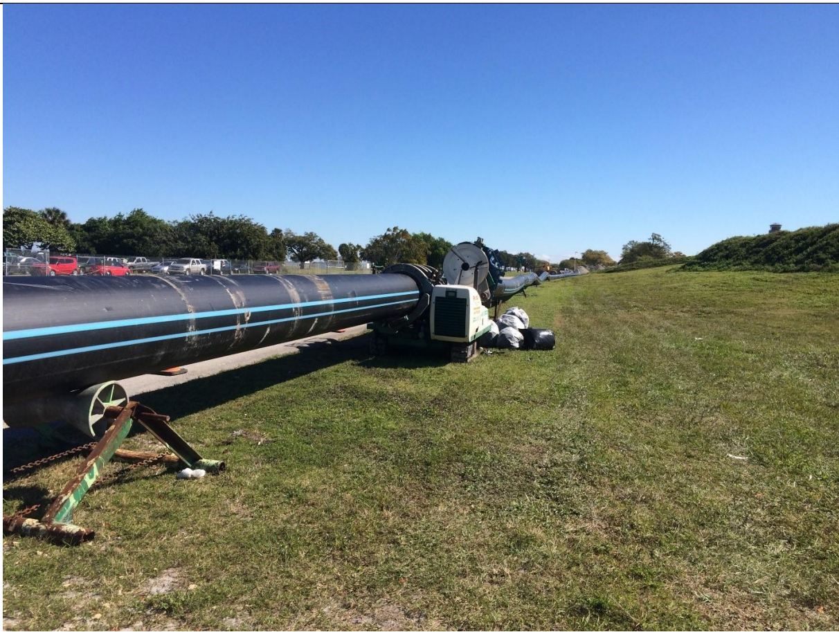
Water main to be installed by HDD
