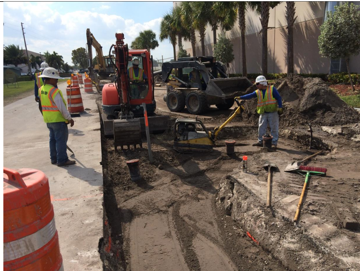
Pavement restoration after water main installation
