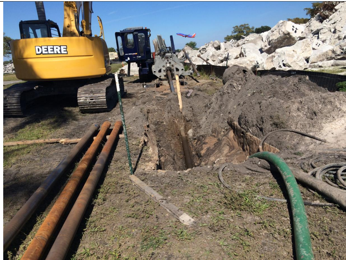
HDD Machine in operation for water main installation
