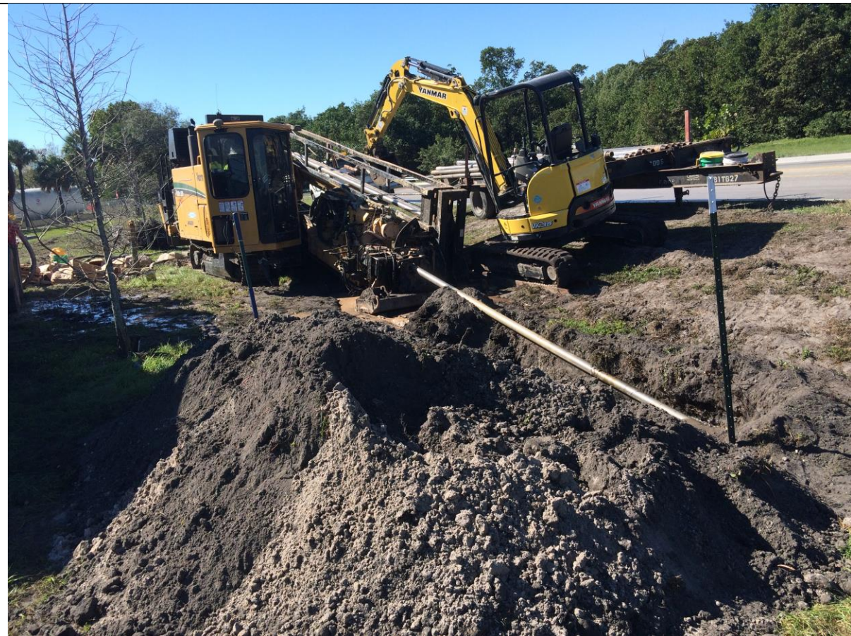
Horizontal Directional Drilling Equipment for pipe installation
