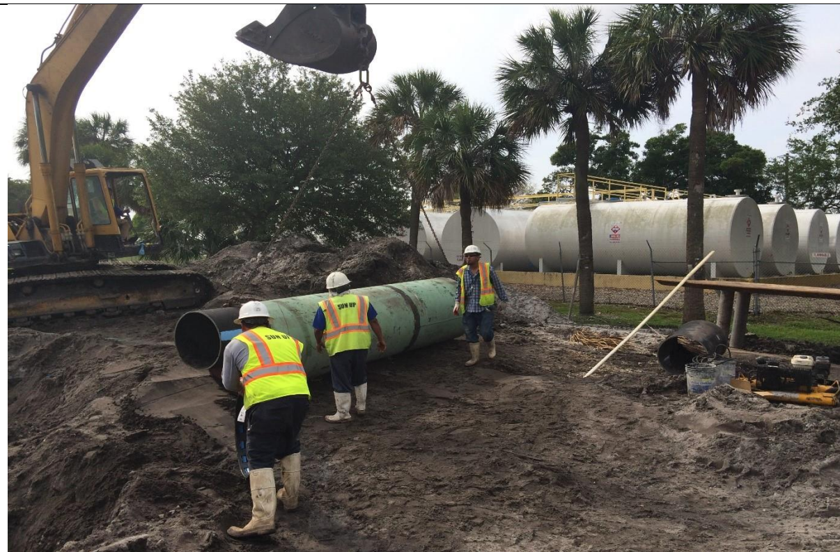
Contractor crew accommodating pipe to be installed.
