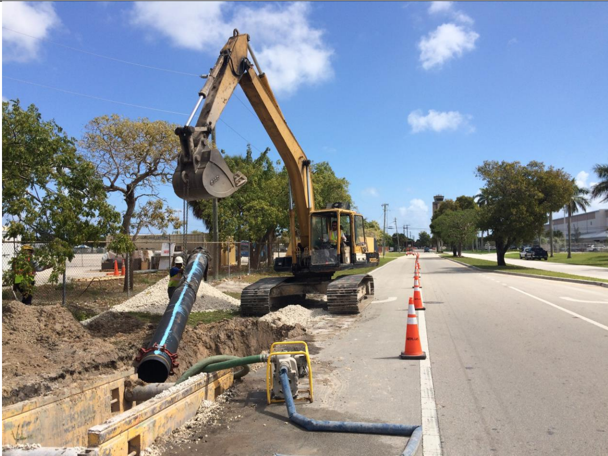
Water Main Installation at Lee Wagener Boulevard
